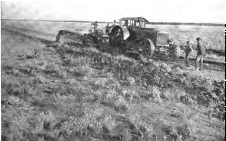
FIG 75.—Building Lateral in Montana with Elevating Grader.
